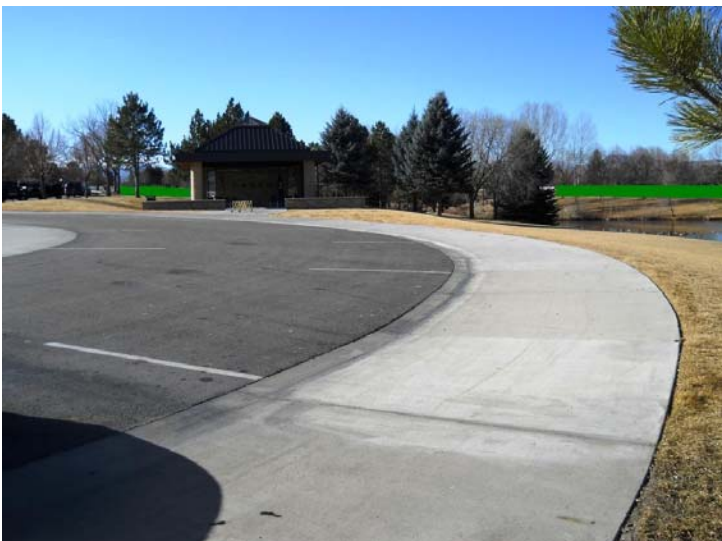
View toward Shelter at tree line – Note droppings
